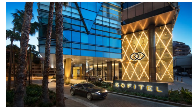
Sofitel Sydney Darling Harbour exterior
